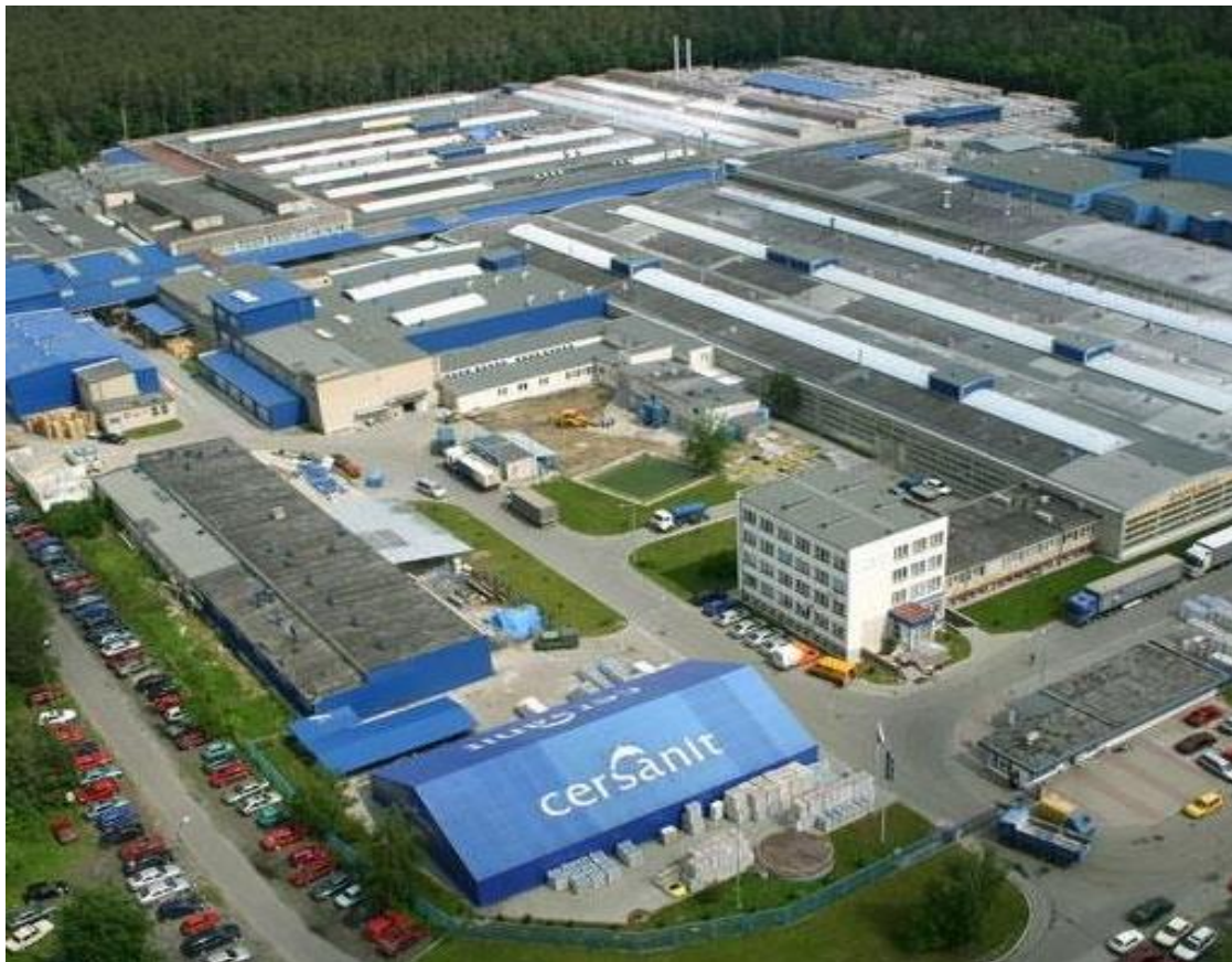
Fig. 1. Cersanit manufacturing plant located in Krasnystaw (Poland).
